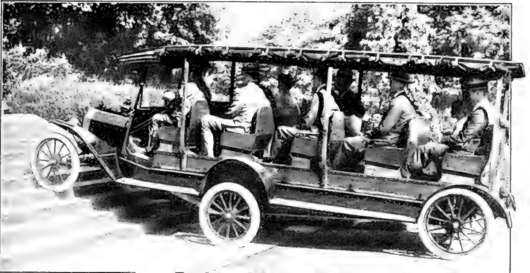
Above: An ingenious six-wheeled automobile, with the body mounted flexibly on the frame at two points (Autoport System)
